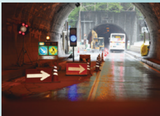
Service and utility tunnels, construction sites
